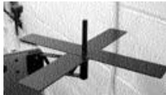
B Install bracket and tape Tray
