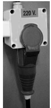
E- Wire the blue plug 220 Volts single phase 15 Amps
